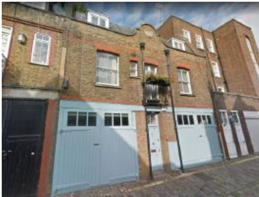
Photograph 4: Front elevation of 19 Wigmore Place
